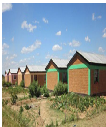
SMA building project in Twafwane, Zambia which has been supported by FoA
